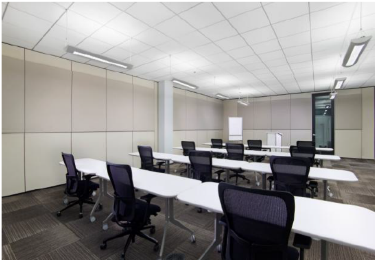
Figure 7. Armstrong Industries DC Lighting Infrastructure (Courtesy of Armstrong, 2009)
